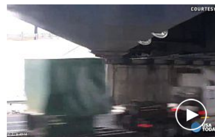
Watch trucks slam into low hanging bridge
